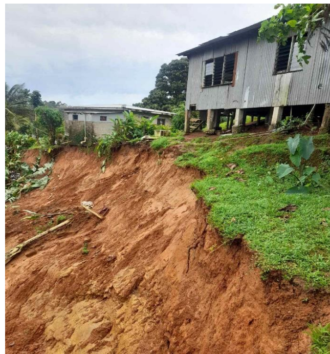
Figure 6h: Landslide from heavy rainfall (Suva – Wailoku)
